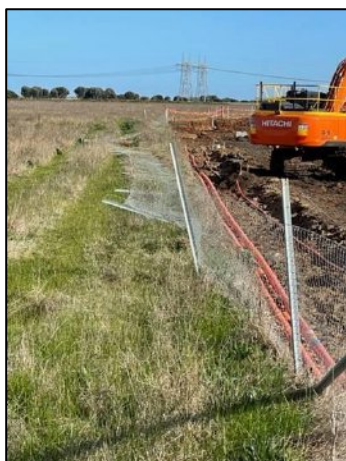
Plate 36. Fence damage from adjoining construction on the north-western boundary (AES 10/08/2022).
