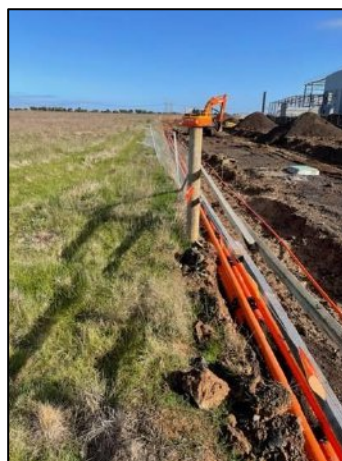
Plate 37. Section of fence that have been damaged during infrastructure installation (AES 10/08/2022).
