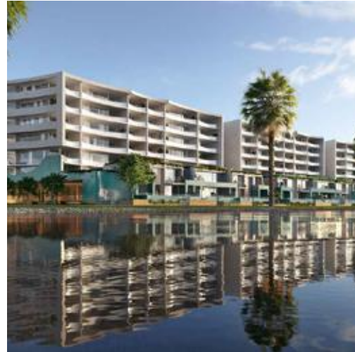
21 HONEYSUCKLE DRIVE - The LUME project comprising 154 apartments. Construction has commenced on the 7,292 square metre parcel of prime waterfront land following a marketing campaign in October 2017 that was well received by purchasers.
