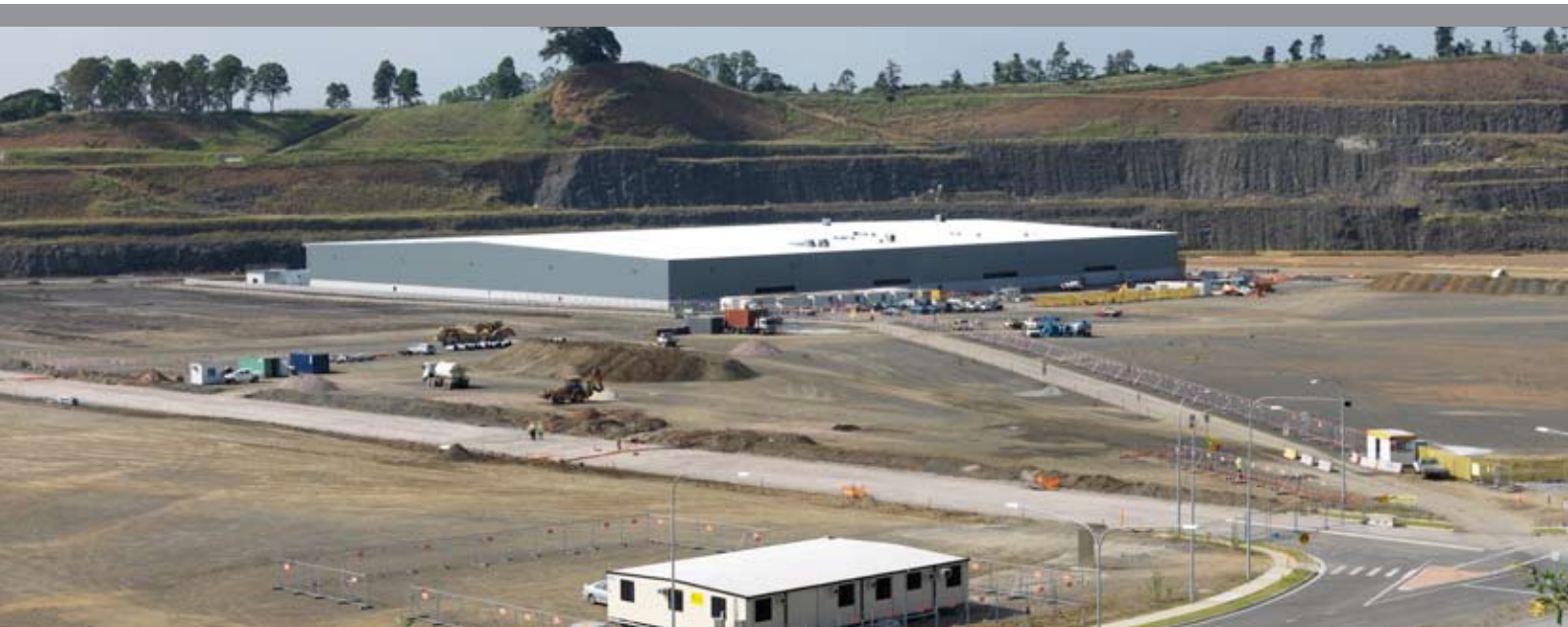
Greystanes Industrial Estate, Reconciliation Road, Greystanes, NSW
