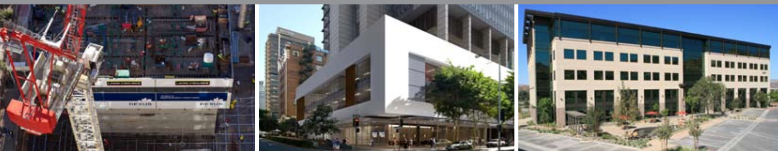
L to R: Construction underway at 123 Albert Street, Brisbane, QLD; Artist's impression of 123 Albert Street, Brisbane, QLD; Summit Oaks, Valencia, CA
