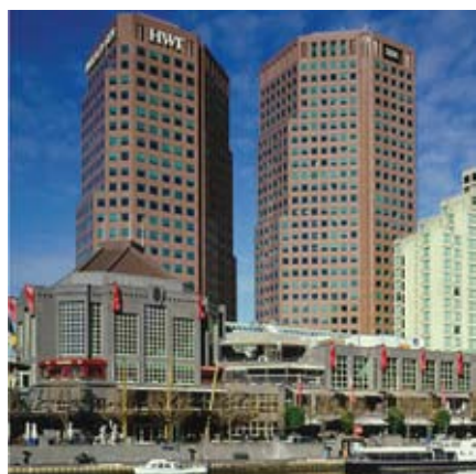
Southgate Complex, 3 Southgate Avenue, Southbank, VIC
