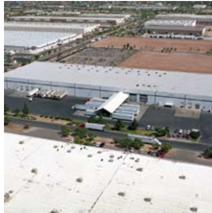
431 North 47th Avenue, Phoenix, Arizona
