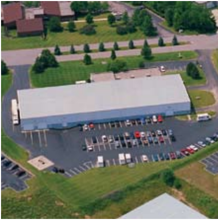
124 Commerce Boulevard, Loveland, Ohio
