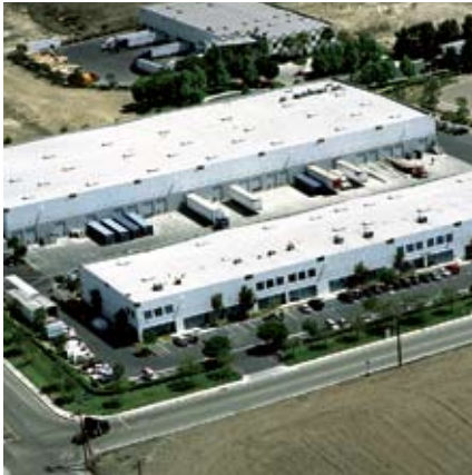
7510-7520 Airway Road, San Diego, California
