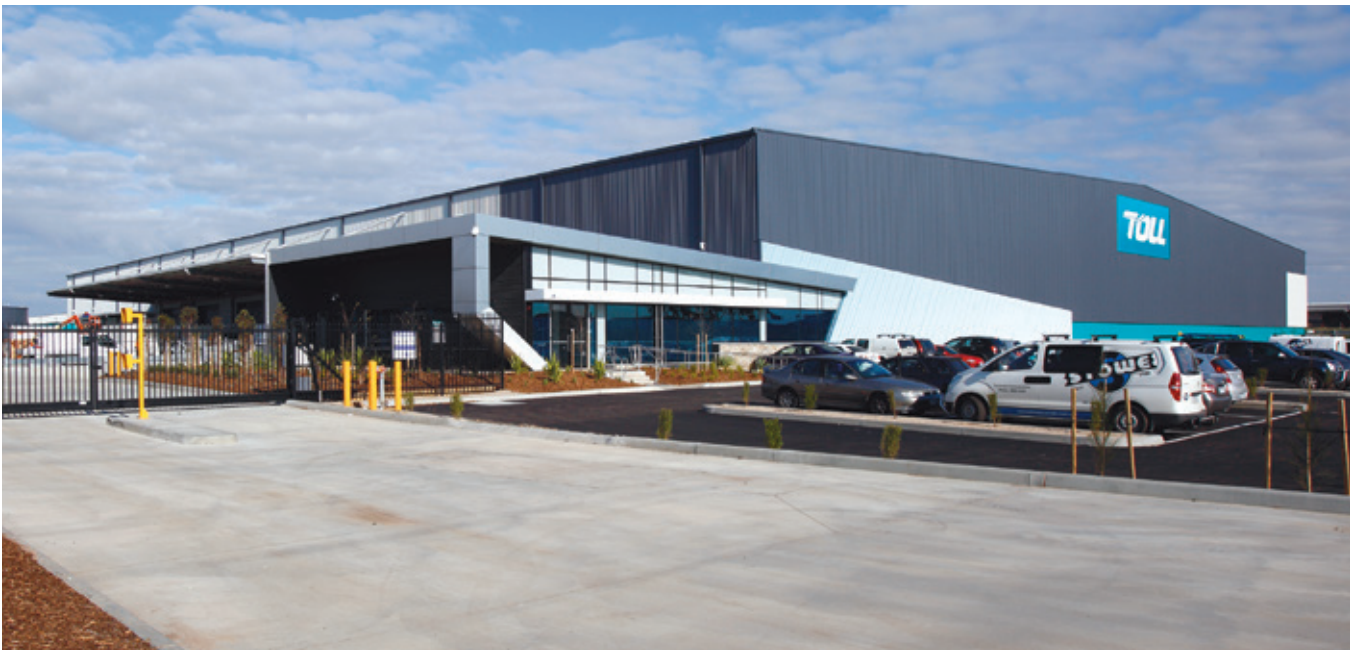
DEXUS Industrial Estate, 27 Distribution Drive, Laverton North, VIC
