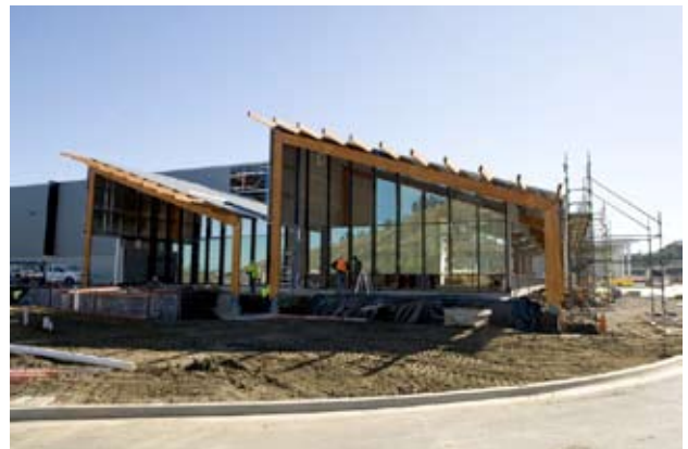
Solaris development at Greystanes, NSW
