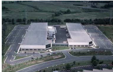
Beaumeade Telecom - Beaumeade Circle, Ashburn, Virginia
