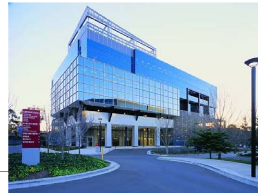
Building C, 11 Talavera Road, North Ryde
