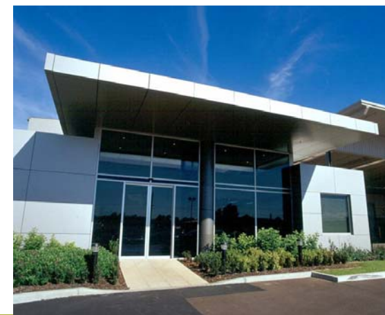
52 Holbeche Road, Arndell Park
