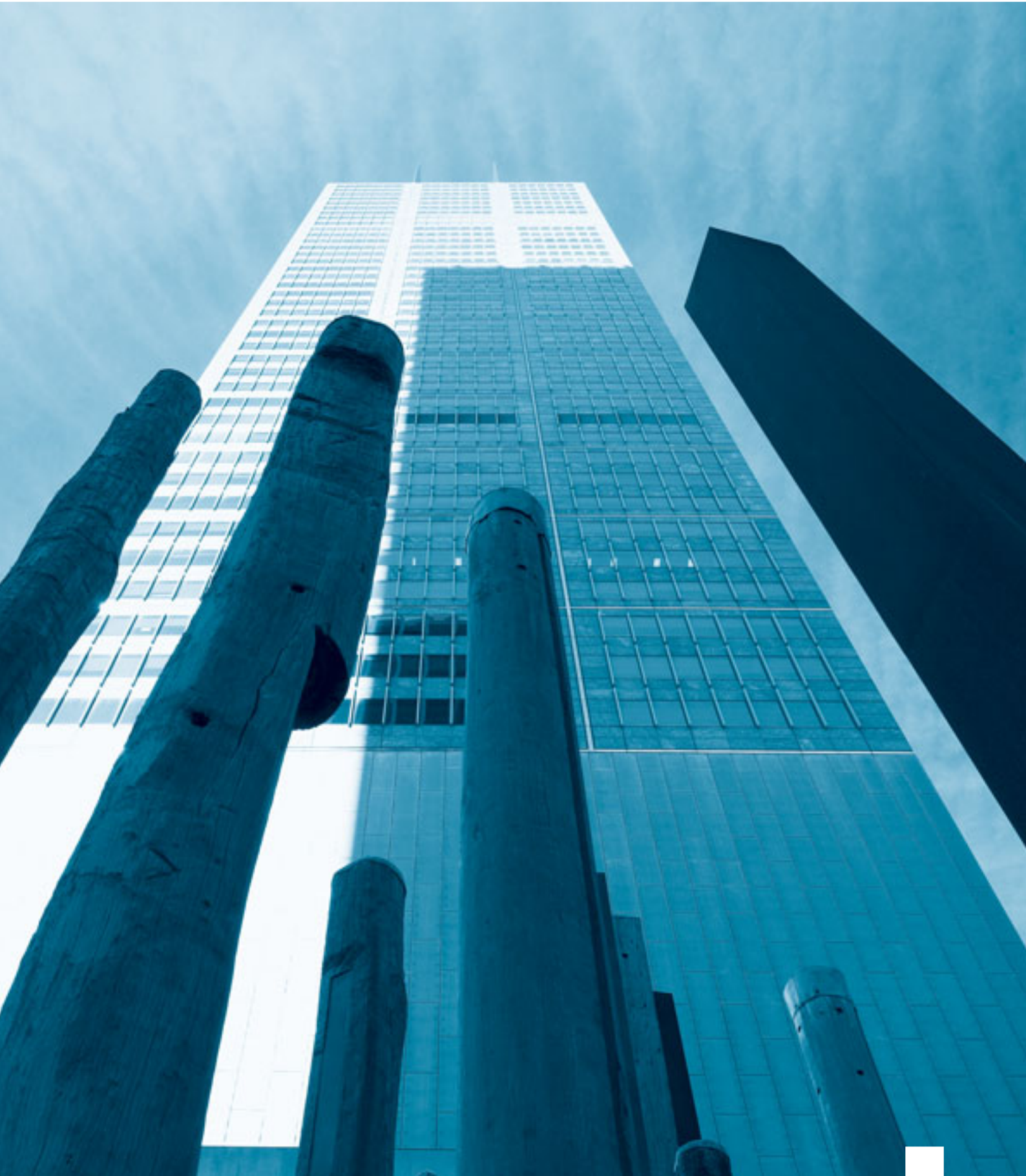
Governor Phillip Tower and Governor Macquarie Tower Office Complex, 1 Farrer Place, Sydney NSW (Photo provided by Hamilton Lund of Visual Eyes International)
