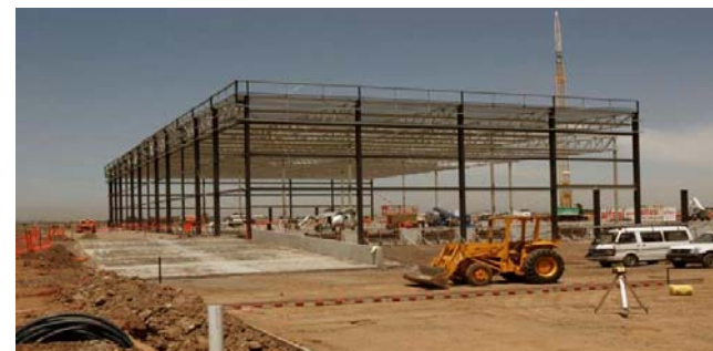
Construction of Coles Myer facility, Laverton
