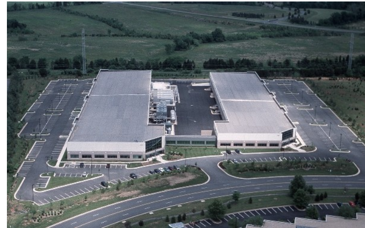
Beaumeade Telecom - Beaumeade Circle, Ashburn, Virginia
