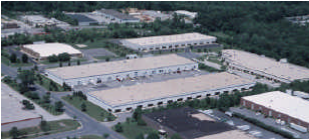
Bristol Court Bristol Court, Jessup, Maryland
