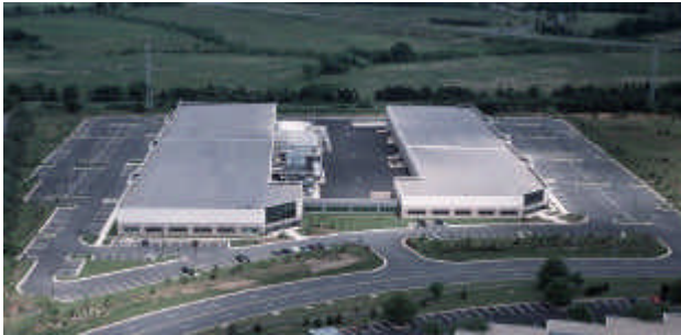
Beaumeade Telecom Beaumeade Circle, Ashburn, Virginia
