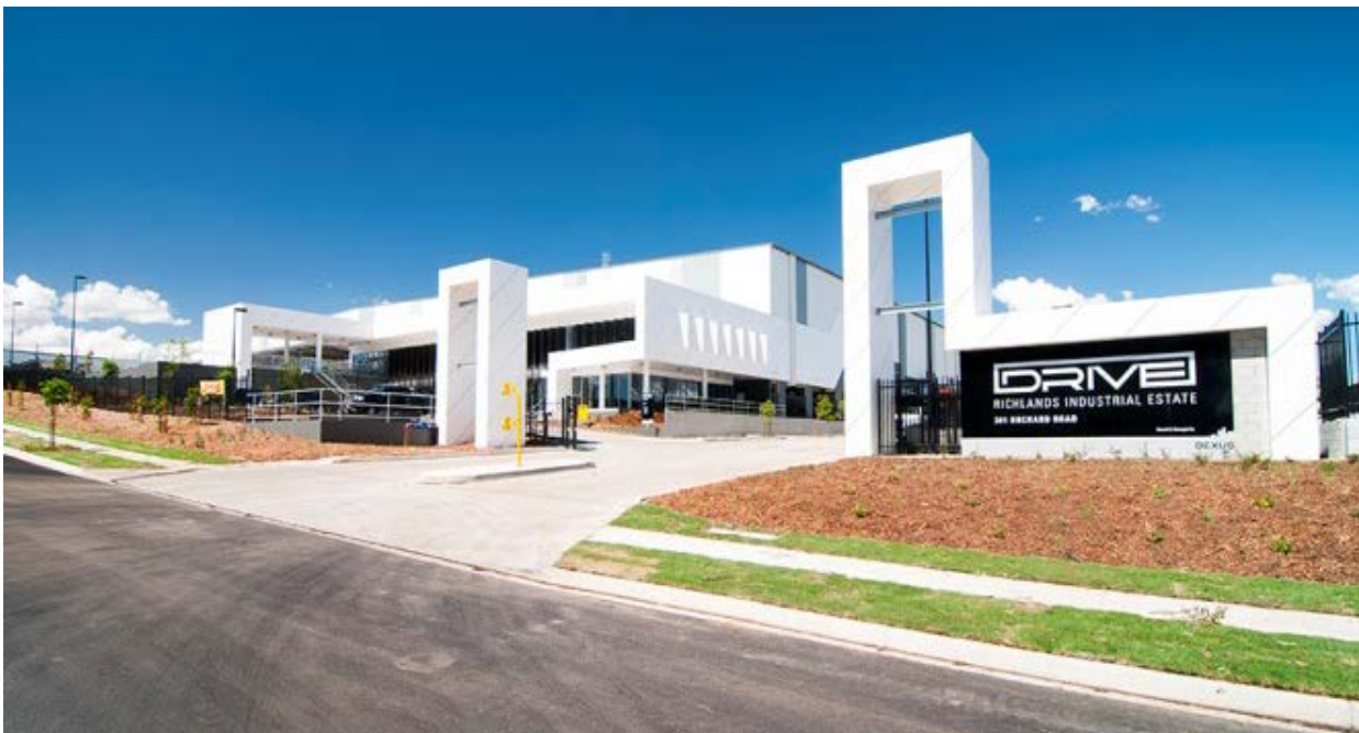
Drive Industrial Estate, Richlands
