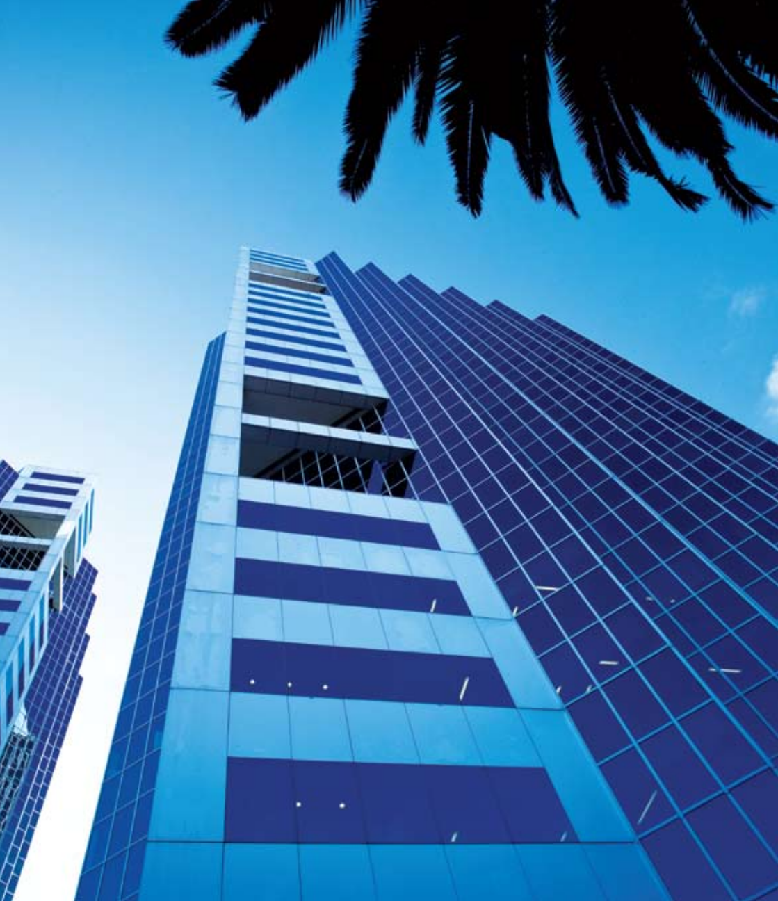
The Zenith, Pacific Highway, Chatswood, NSW
