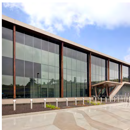
Quarry Industrial Estate, 6 Bellevue Circuit, Greystanes
