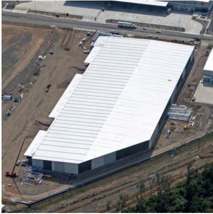
Quarry Industrial Estate, 3 Basalt Road, Greystanes
