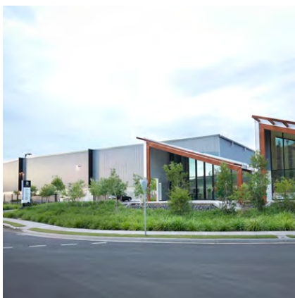
Quarry Industrial Estate, 8 Basalt Road, Greystanes
