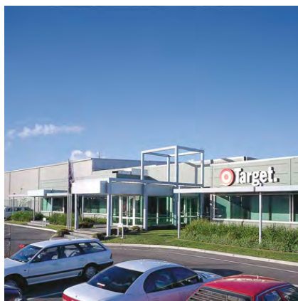
Target Distribution Centre, 30-68 Taris Avenue, Altona North
