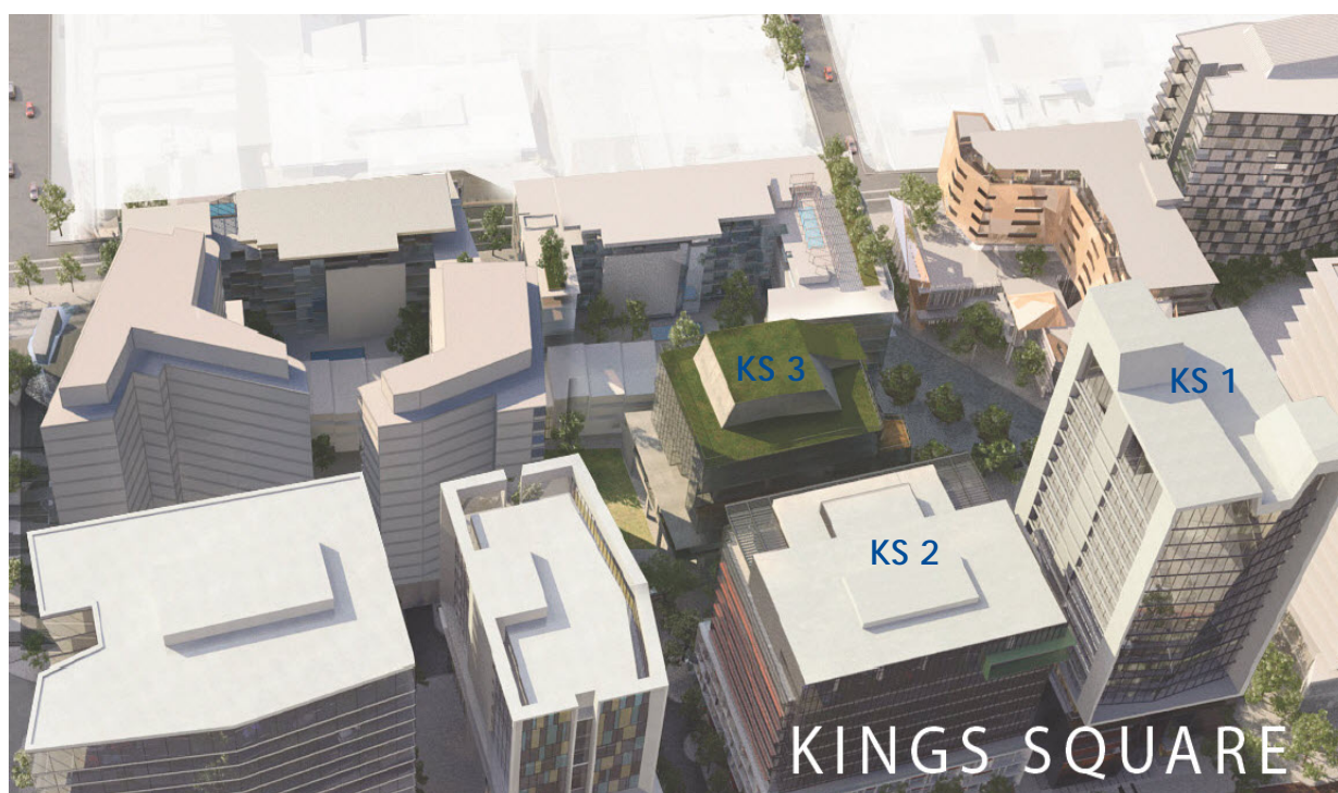
KS1, KS2, KS3 Office properties that DXS and DWPF are acquiring through Kings Square transaction.
