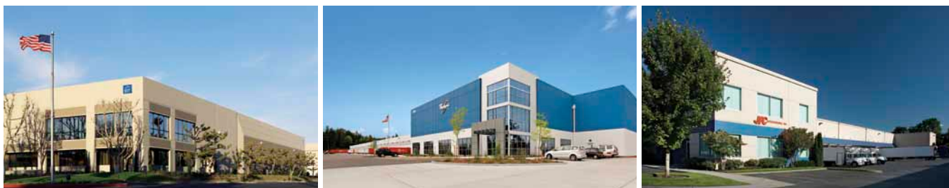
L to R: 1777 S Vintage Avenue, Ontario, CA; 19700 38th Avenue East, Spanaway, Seattle, WA; Riverbend Commerce Park, 8005 South 266th Street, Kent, WA
