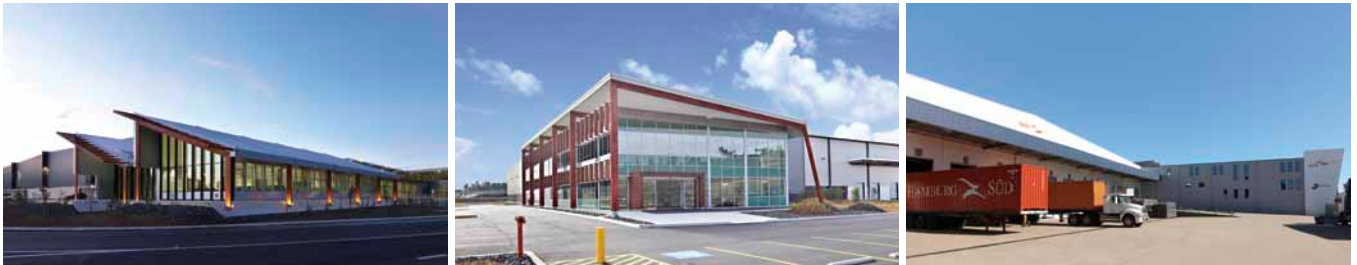
L to R: 8 Basalt Road and 2-6 Basalt Road, Greystanes, NSW; 2-4 Military Road, Matraville, NSW
