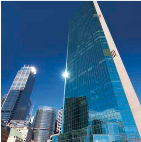
Governor Phillip Tower, 1 Bligh Street, Gateway, Sydney, NSW
