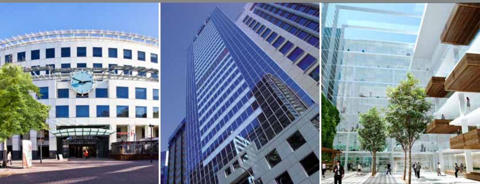
L to R: Garema Court, 140-180 City Walk, Canberra, ACT; 45 Clarence Street, Sydney, NSW; Artist's impression of Flinders Gate Complex, Melbourne, VIC
