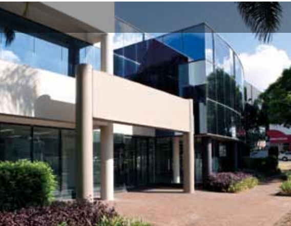
Centrewest Industrial Estate, 108-120 Silverwater Road, Silverwater, NSW
