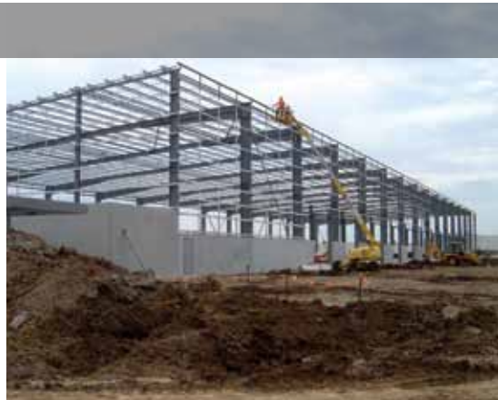
Loscam development, DEXUS Industrial Estate, Boundary Road, Laverton North, VIC
