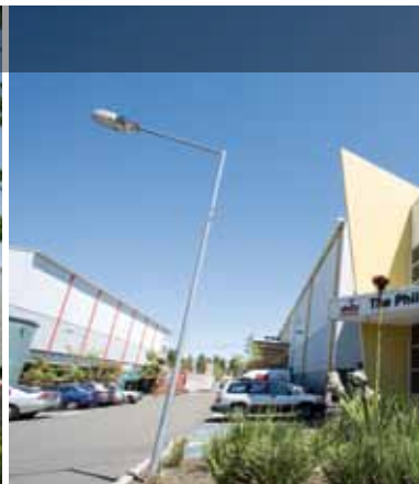
1 Foundation Place, Greystanes, NSW
