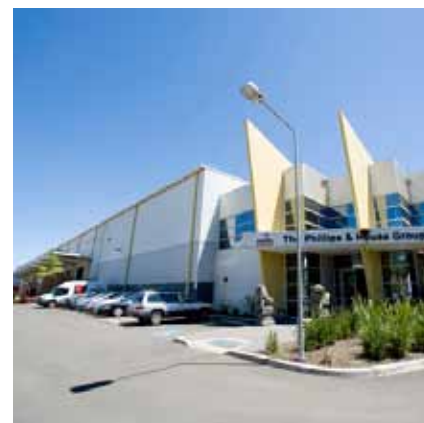
1 Foundation Place, Greystanes
