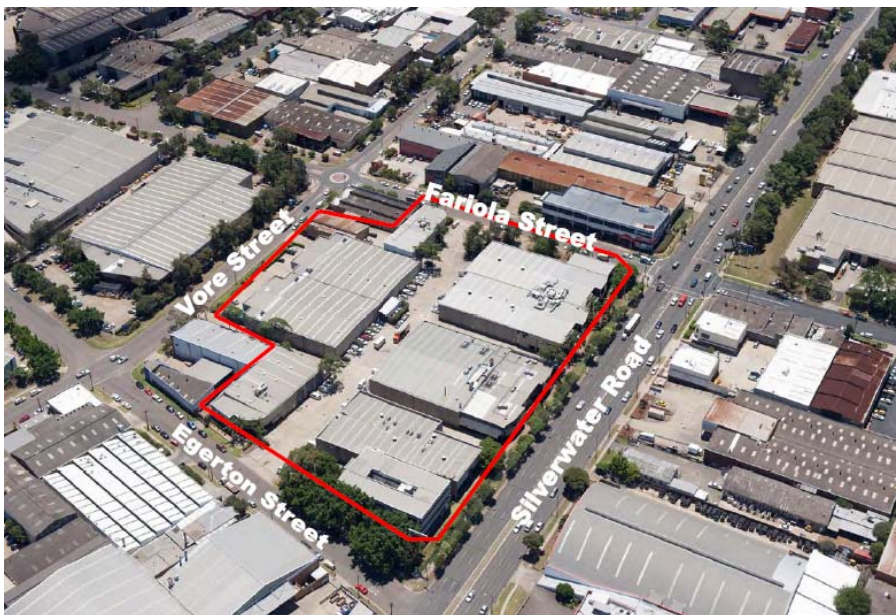
Aerial view of 108-120 Silverwater Road, Silverwater NSW
