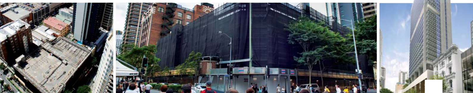
Above: Construction is underway at 123 Albert Street, Brisbane QLD (left and centre) and an artist's impression of the completed office tower (right)
