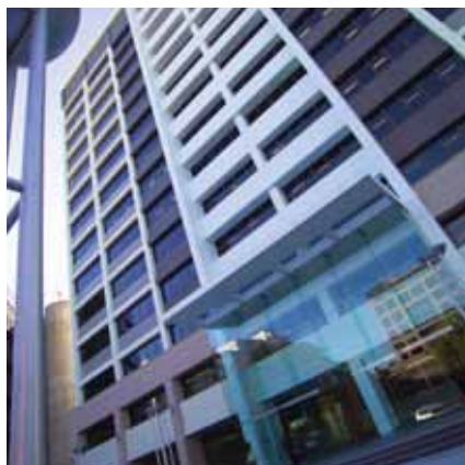
Ferguson Centre 130 George Street Parramatta, NSW
