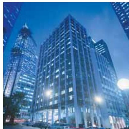
O'Connell House 15–19 Bent Street Sydney, NSW
