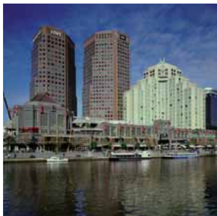
Southgate Complex 3 Southgate Avenue Southbank, VIC
