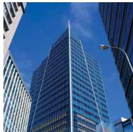
Lumley Centre 88 Shortland Street Auckland, NZ
