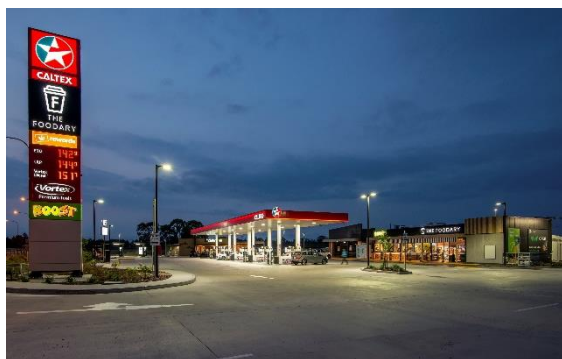
Brisbane Airport Link Service Centre
