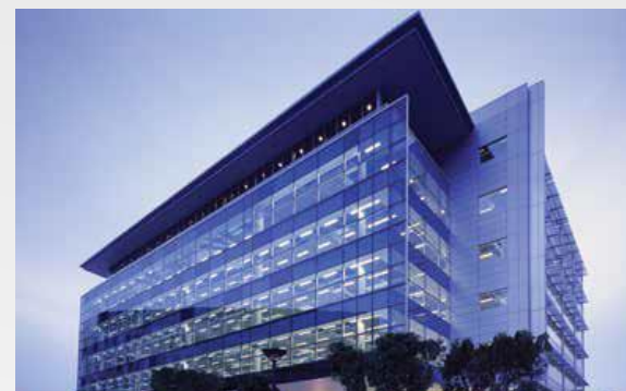
Building A, 1 Homebush Bay Drive, Rhodes NSW
