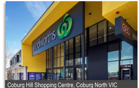
Coburg Hill Shopping Centre, Coburg North VIC
