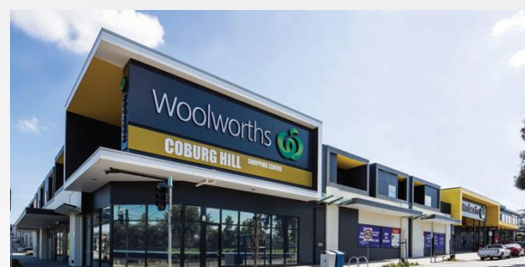
Coburg Hill Shopping Centre, Coburg North VIC
